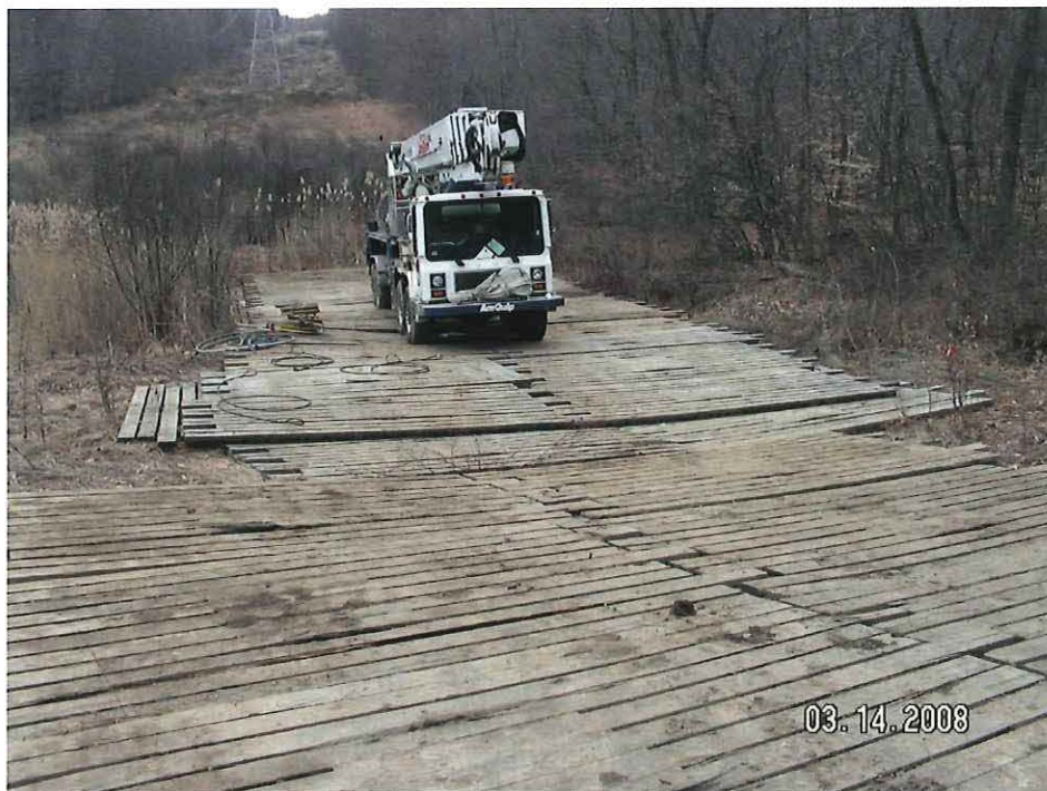
Photograph Number 2- Typical Mats used in Wetlands near Tower and along ROW
