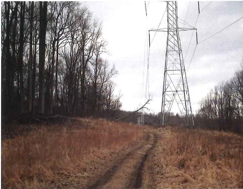
Photograph Number 5- Tree on Transmission Wire
