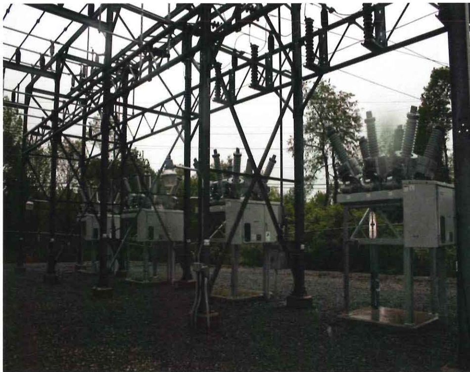
Photograph Number 4- New Breakers Added to Existing Substation
