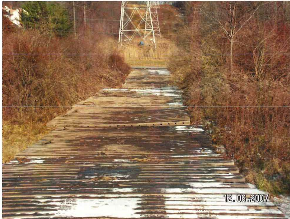
Photograph Number 3- Typical Mats used in Wetlands near Tower and along ROW
